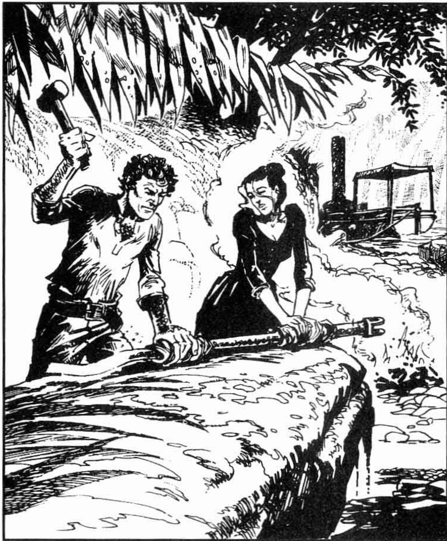
It was a week of back-breaking and dangerous work.
